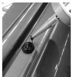
4. Locate rail on top and place M8 stainless bolts through the holes.
